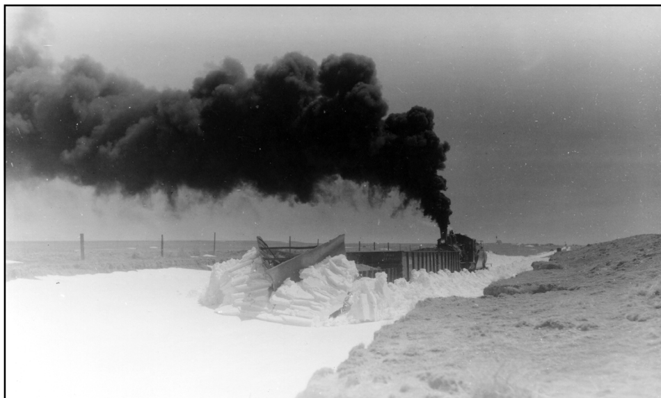
Otto Perry made a sojourn to Keota, Colorado where he caught the last Burlington ten-wheeler (4-6-0) number 919, pushing a wedge snowplow through a snow filled cut. The prairie was clear of snow by April 15, 1955, when this view was taken.
